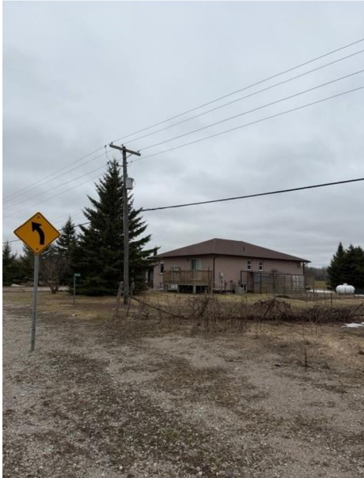
Existing house on severed lands
